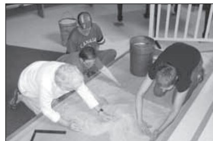
Laying the base
