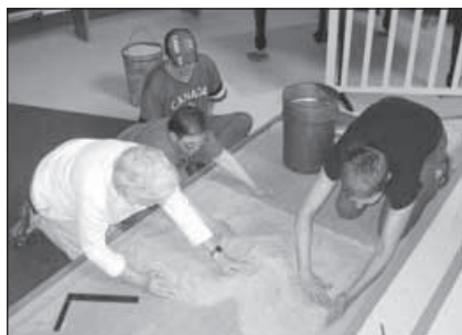
Laying the base
